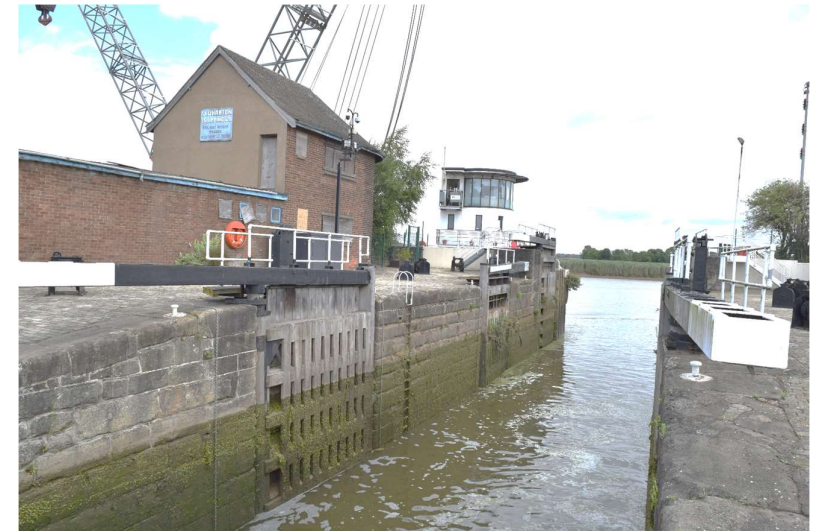
Figure NTS7: View east along Keadby Lock [1005204; 1342734] at its exit to the River Trent, adjacent to the Waterborne Transport Offloading Area
